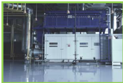
ZK1200 Gas Turbine Set
